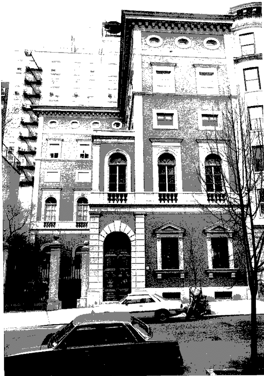
Fig. 24. Ernesto and Edith Fabbri House, 7 East 95th Street (1914).
