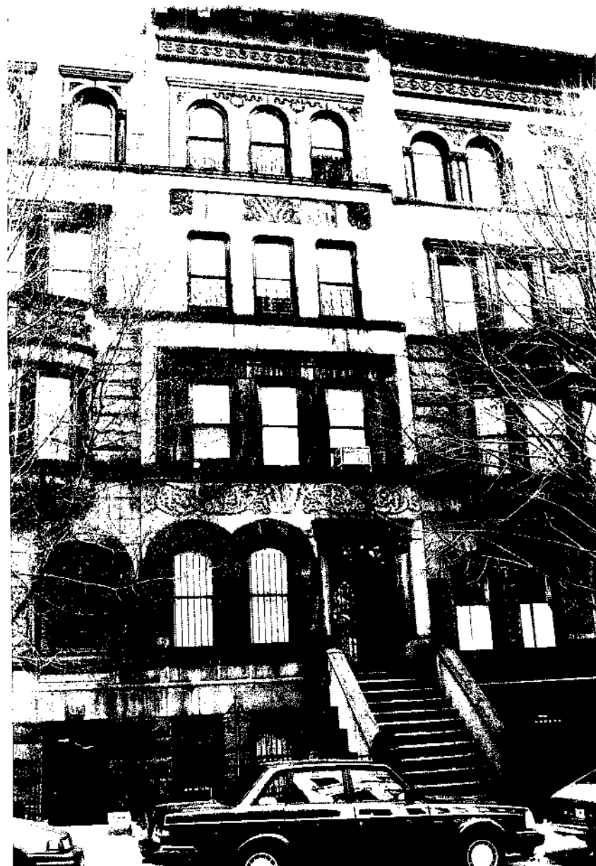
Fig. 9. No. 22 East 93rd Street (1893).
