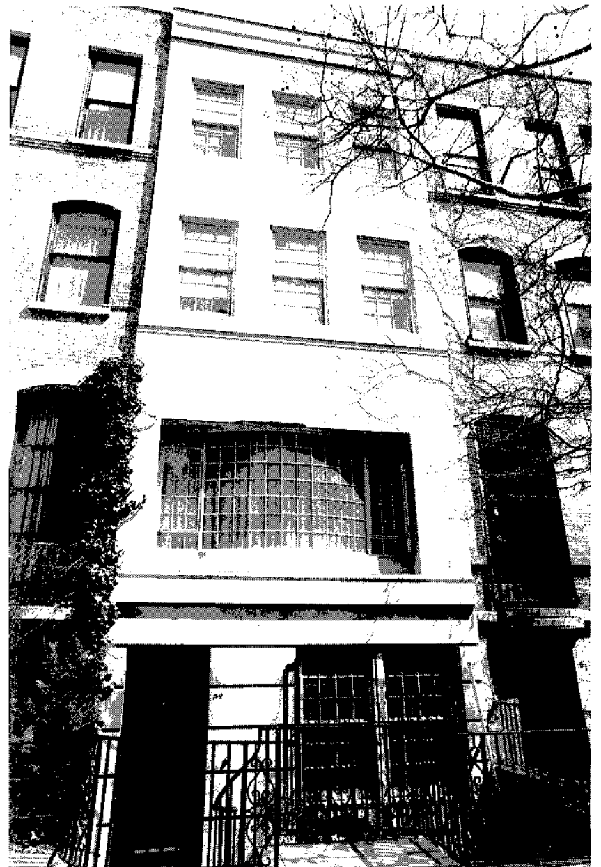
Fig. 35. No. 59 East 93rd Street (1937).
