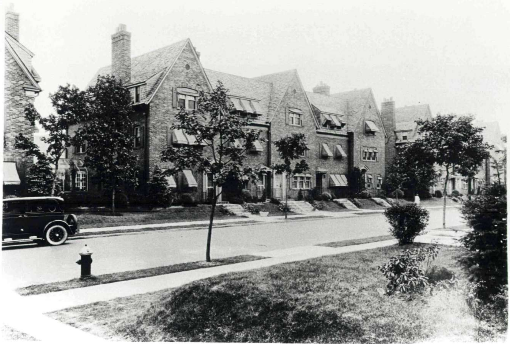
Fig. 27. Garden Homes (C.F. & D.E. McAvoy, 1925), east side of 87th Street between 35th and 37th avenues, c. 1926.
